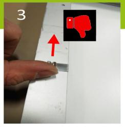
Test a clip on the solar panel with the logo side downwards. It should be so securely fastened that it's nearly impossible to push upwards. If it is possible to slide it upwards, then use a pliers to adjust the clips on the logo side untill it is okay. Put 7 clamps (logo visible) per black BirdBlocker and at least 2 per small piece that can easily be cut to size.
