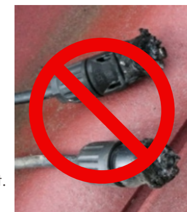
Example of improper cable installation 15
