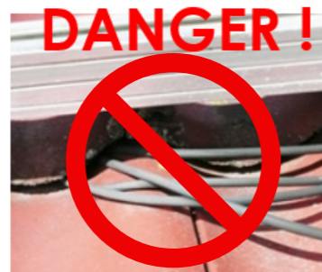
Improper cable installation 13
