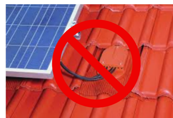
Example of improper cable installation 14
